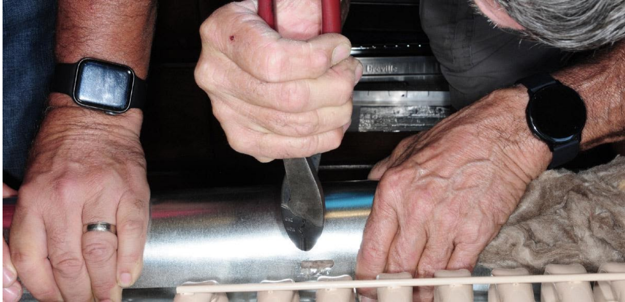
Closing the housing for the heating elements takes some finesse, or a bunch of extra hands.
